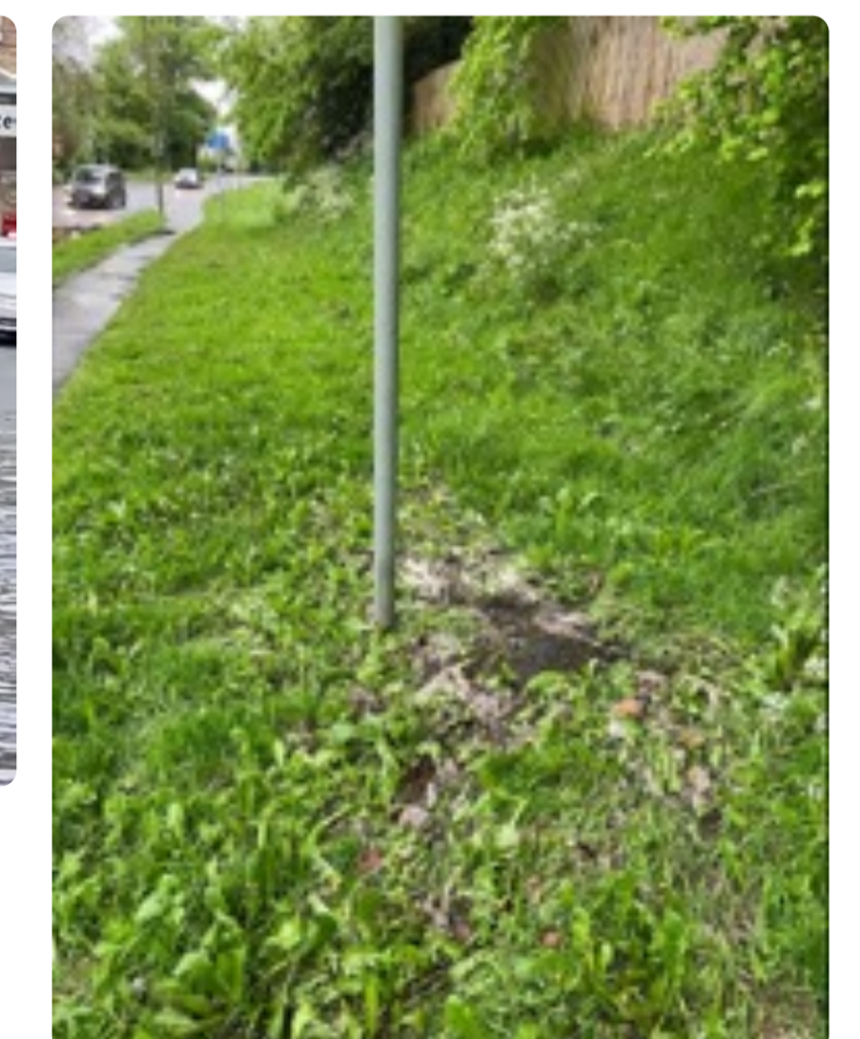
Photo of sewerage leak on London Road
