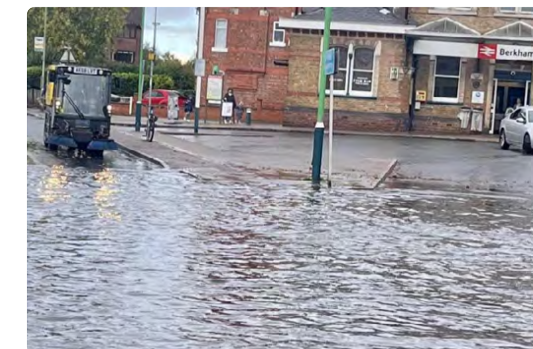
Photo of flooding on Station Road
