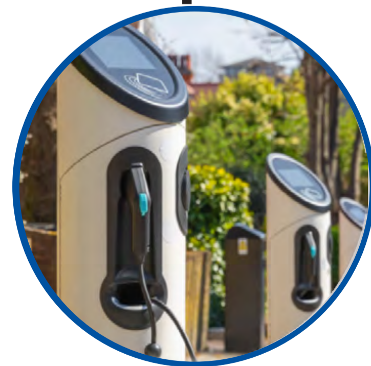
Electric charging points
